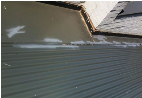
Figure 1. Irregular faded appearance of touch-up paint on roof flashing and roofing broad sheet
