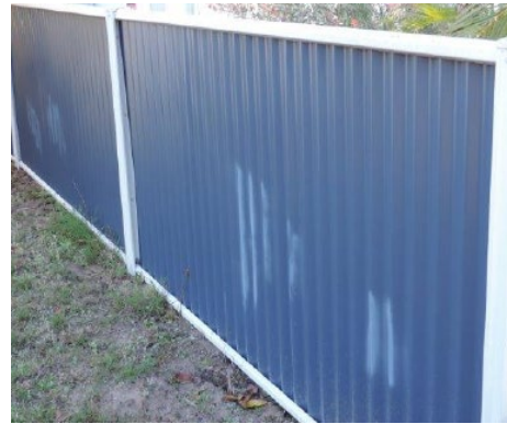
Figure 2. Irregular faded appearance of touch-up paint on fencing panels
